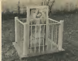
Hammered to pieces by vandals about five years ago, stone now has been framed, set in base of concrete and circled by steel rails.
